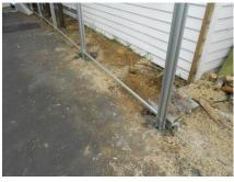
next posts height. Repeat this for all posts. The last panel may be trimmed to suit a specific post centre. *TIP: From our experience we have found that temporarily fitting the rails top and bottom keeps the posts correctly spaced and aligned while concreting the posts into position. Note – You are not necessarily fitting the rails to their final position at this point – they are just acting as spacers and they can be moved to their correct position once concrete has set off.*
